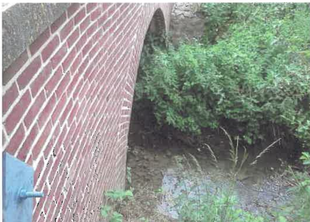
Figure 14 photo ruisseau St Pierre (rapport de stage VNF 2011 C. Demol)
